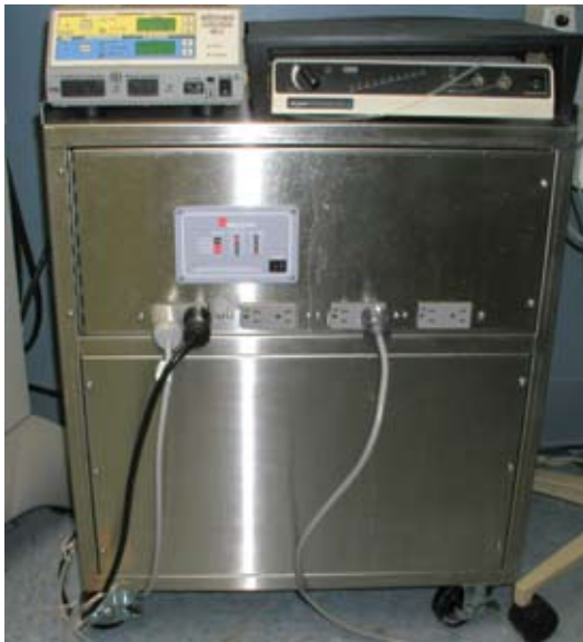
FIGURE 4-3 A back-up power supply was one piece of equipment required for accreditation.
